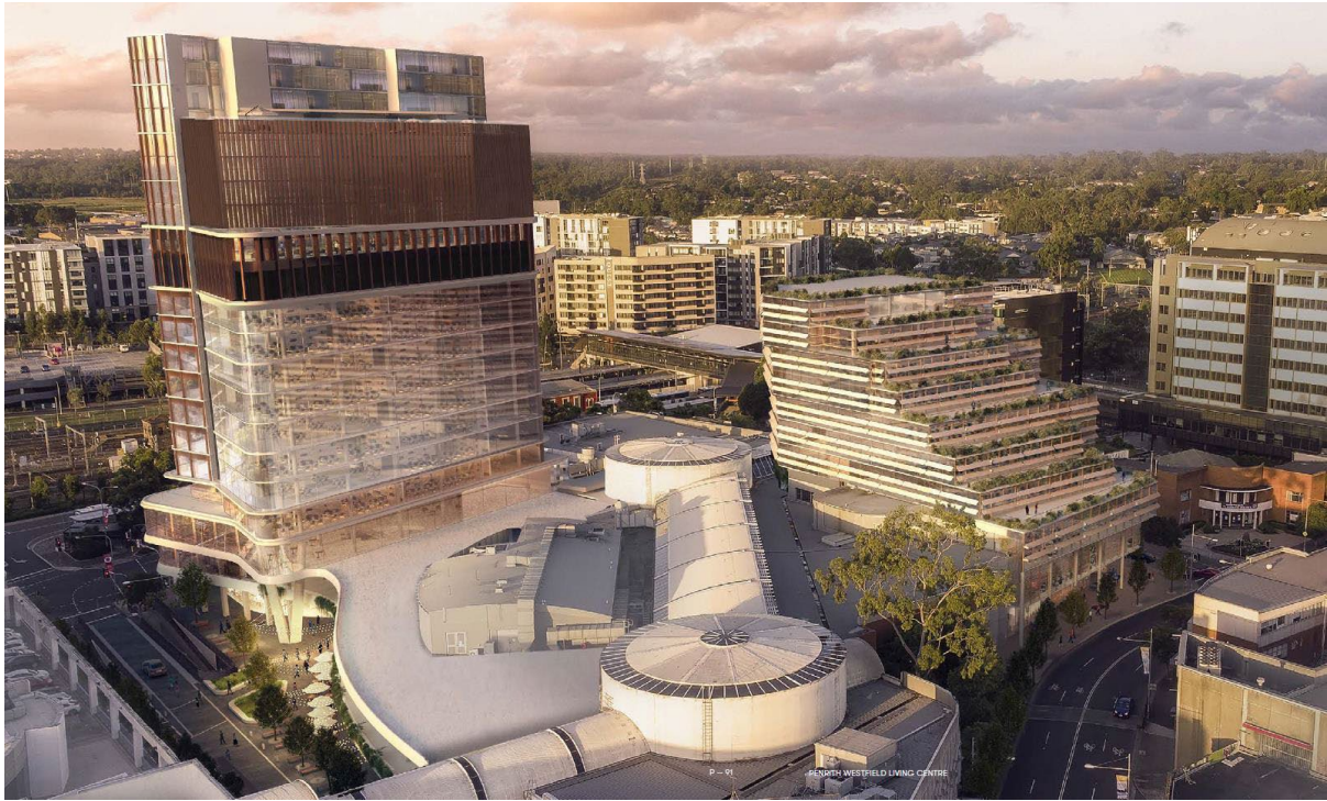
Block A (The Hub) and Block B (Borec House) – View North-east
